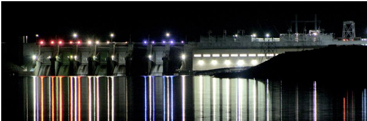
Figure 5 - Little Goose Lock and Dam (Photo: US Army Corps of Engineers)
