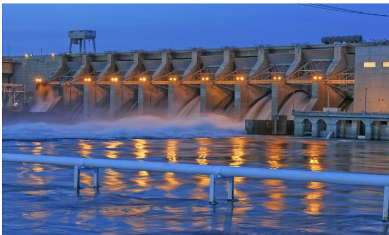
Figure 2 - Ice Harbor Dam (Photo: D.G. Rigg/US Army Corps of Engineers)
