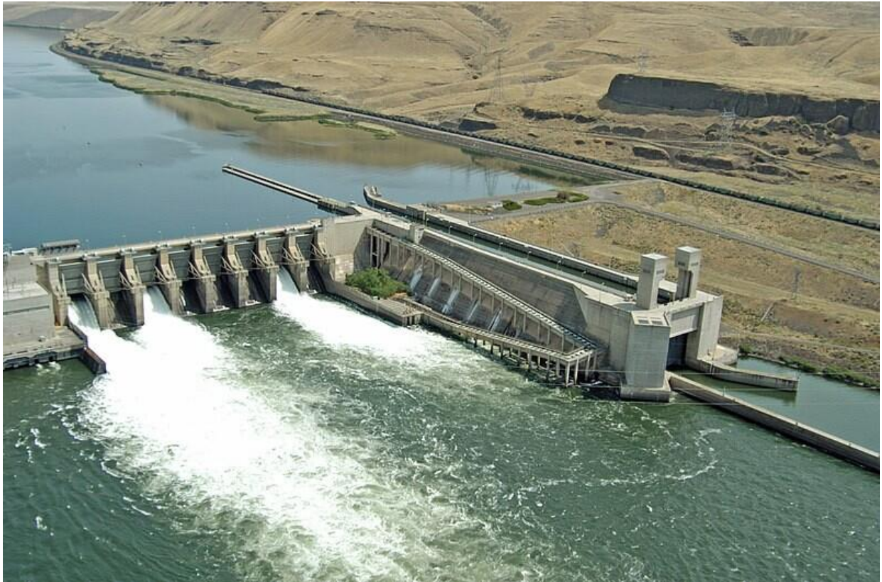
Figure 4 - Lower Monumental Dam fish ladder (Photo: Bonneville Power Administration)
